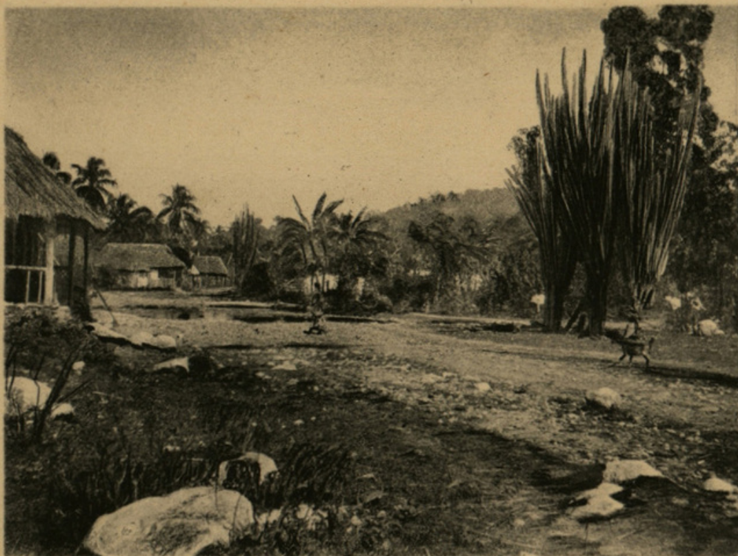
GRESSIER ROUTE DE PORT-AU-PRINCE A LÉOGANE
